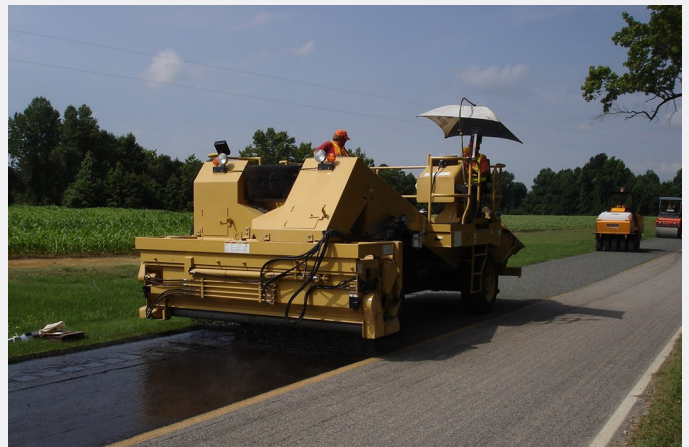
Picture: Chip Seal Construction
